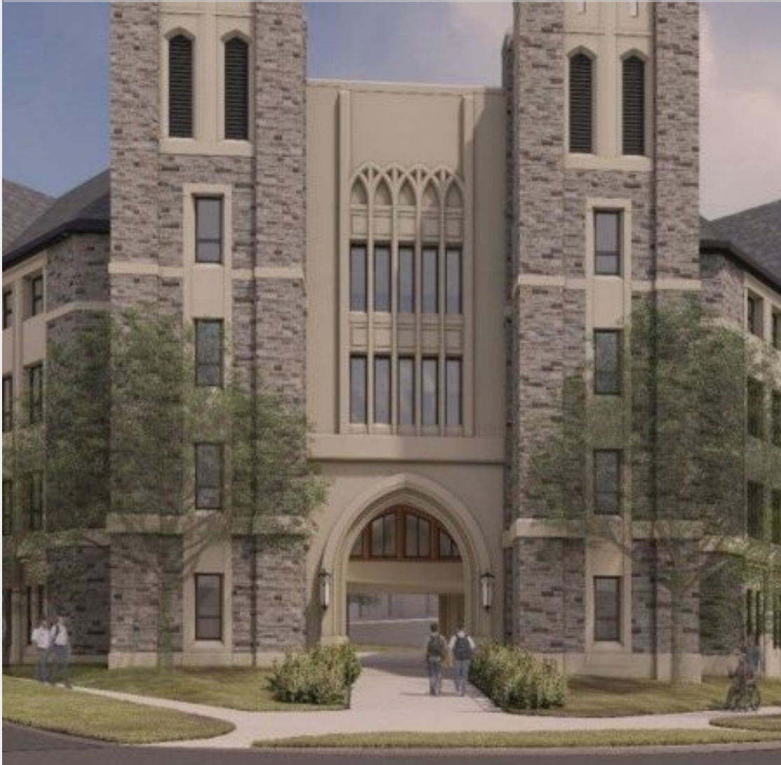
Drillfield to Upper Quad Access Improvements as part of Upper Quad Hall North Capital Project
