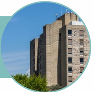
Slusher Hall Repairs
